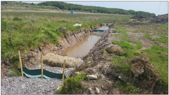
Plate 4-13 Check Dam constructed with stone, straw bales and terram forming a long stilling pond
