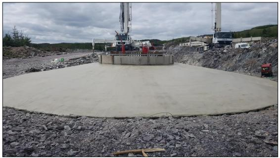
Plate 4-3 Turbine Foundation Poured
