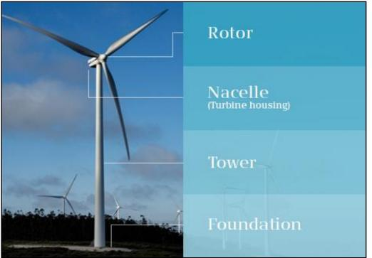
Plate 4-1 Wind Turbine Components.
