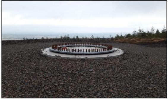
Plate 4-4 Turbine Foundation Back-fill Complete
