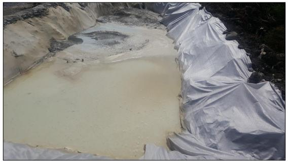
Plate 4-11 Concrete washout area
