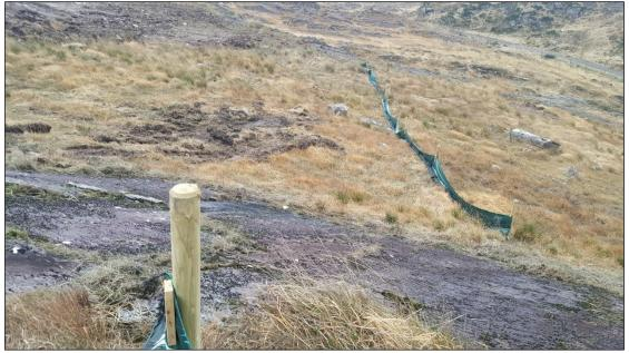
Plate 4-16 Embedded Silt Fence installed down slope of works area
