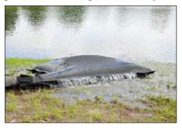
Plate 4-14 Silt Bag with water being pumped through
