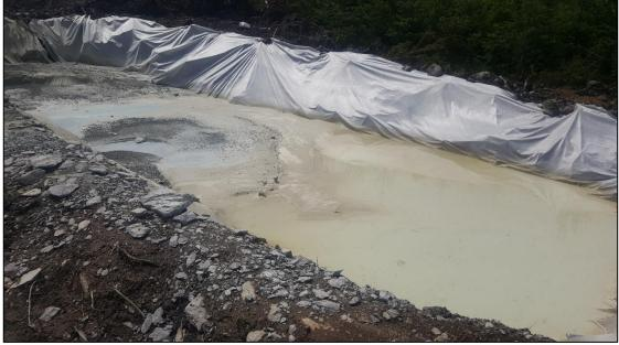
Plate 4-10 Concrete washout area
