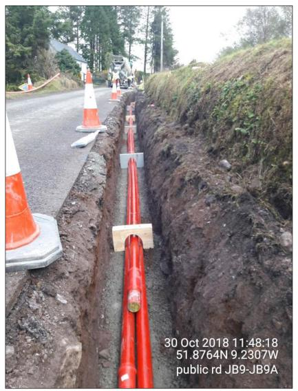
Plate 4-18 Cable Trench with Trefoil Ducting Arrangement
