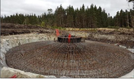
Plate 4-2 Turbine Base 'Anchor Cage'
